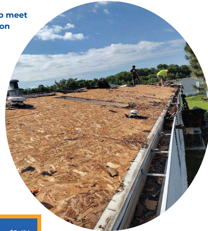
New roof installation
