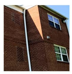
BEFORE AND AFTER: Aging condensing units were replaced with exterior, wall-mounted heat pumps. The abandoned wall penetrations were fully insulated and finished with brick.
